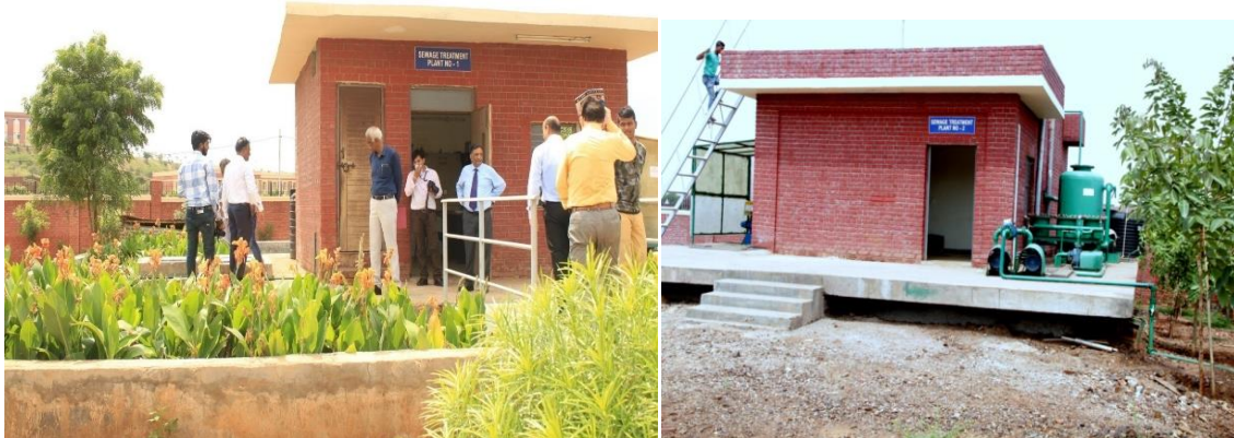
SEWAGE WATER TREATMENT PLANT - 1
